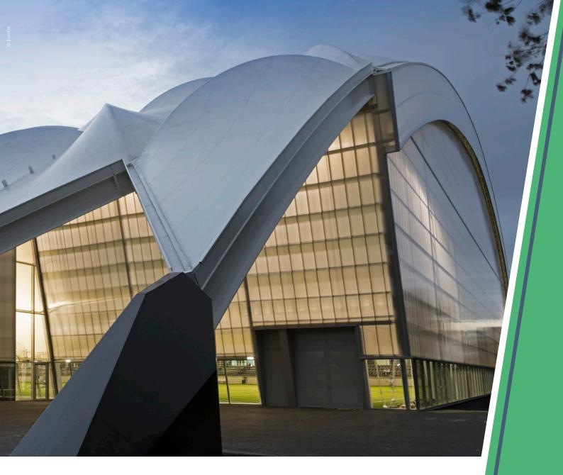
An elegant curved steel frame roof spanning more than 100 metres was clad in tensioned 2mm white PVC fabric and complemented by Danpalon<sup>®</sup> façade panels.
