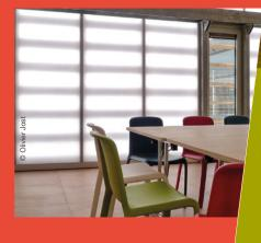
As for the sun-shades, they are positioned in front of the Danpatherm K7. All these elements can be readily separated from each other.
