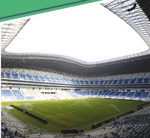
dium, leaving spaces for air to enter and cool the public in a natural way, and continues over the stands with an overhang of up to 50 meters. To build it, they used Building Information Modeling, BIM, a modeling technology which allows for design the structure and allowing to know exactly the materials, locations and virtually exact amounts needed for construction.
