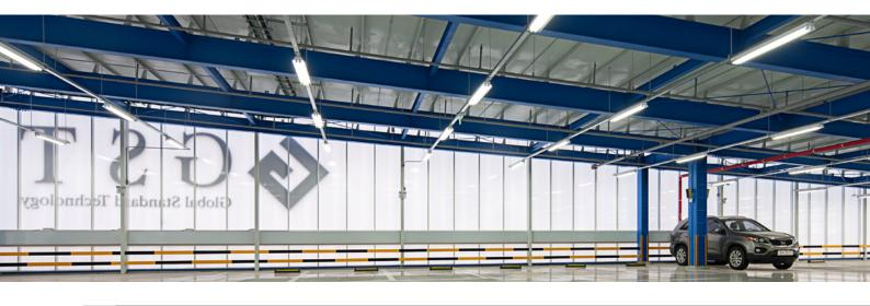
By gently diffusing the outside light and protecting the GST workforce from the effects of direct sunlight, the façade has helped increase efficiency and safety in the workplace while also helping to save energy, by reducing the amount of artificial lighting required along with associated CO<sub>2</sub> emissions.
