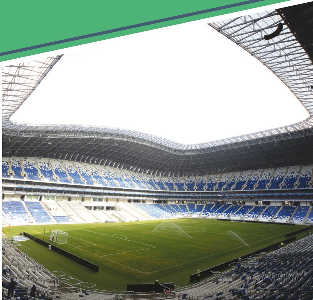
dium, leaving spaces for air to enter and cool the public in a natural way, and continues over the stands with an overhang of up to 50 meters. To build it, they used Building Information Modeling, BIM, a modeling technology which allows for design the structure and allowing to know exactly the materials, locations and virtually exact amounts needed for construction.
