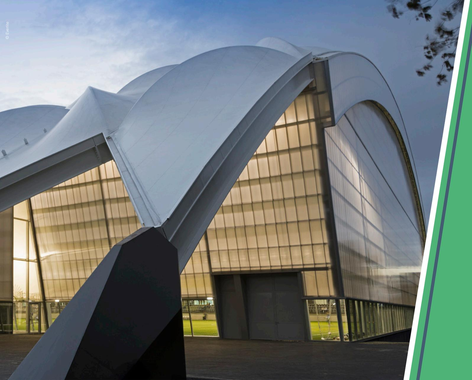
An elegant curved steel frame roof spanning more than 100 metres was clad in tensioned 2mm white PVC fabric and complemented by Danpalon® façade panels.
